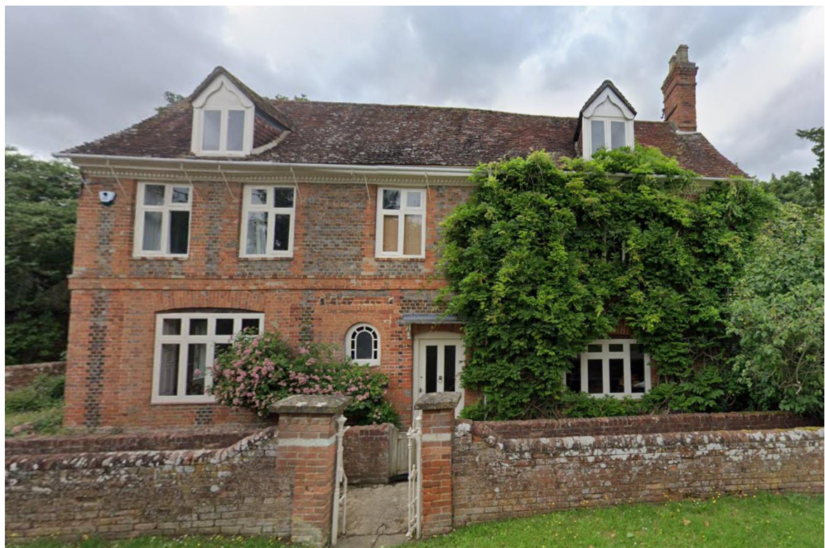
Figure 3.5 - Sunningwell House © Google Maps
