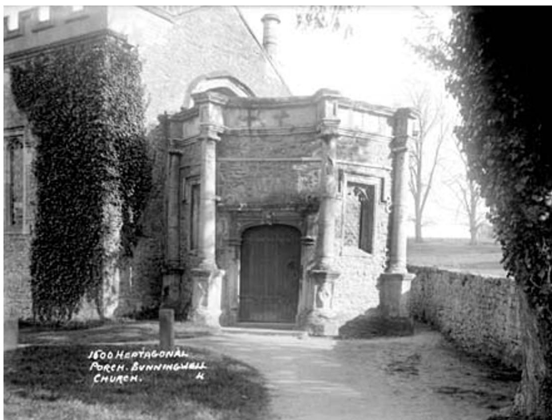
Figure 3.12 - The seven-sided Jewel Porch at St. Leonard's Church Sunningwell – believed to be unique and the first ecclesiastical building to combine Gothic and Renaissance styles.
