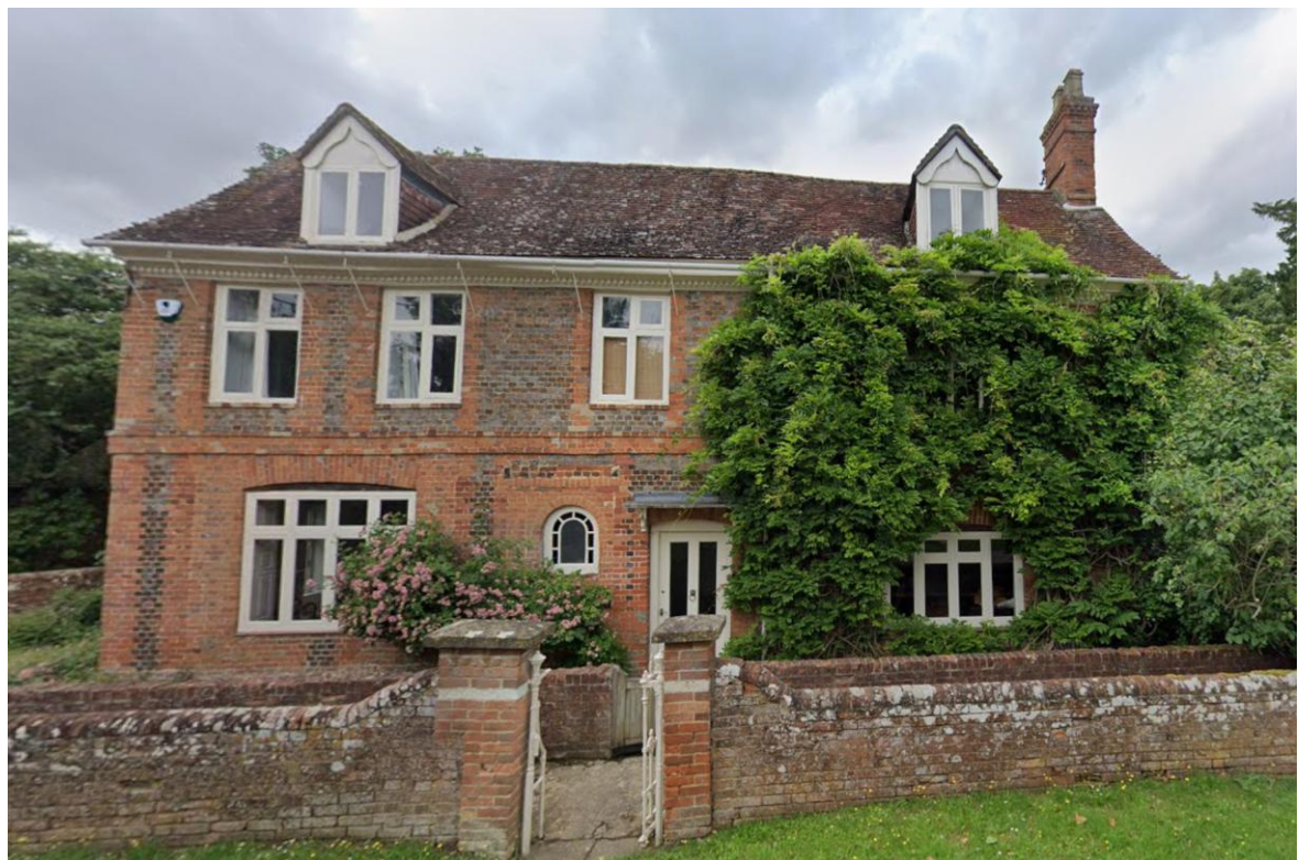
Figure 5.10 - Sunningwell House © Google Maps
